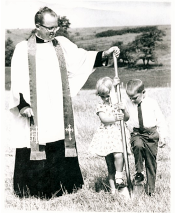
Breaking ground on Dopp St., July 31, 1966
