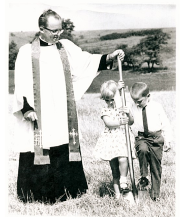
Breaking ground on Dopp St., 1966
